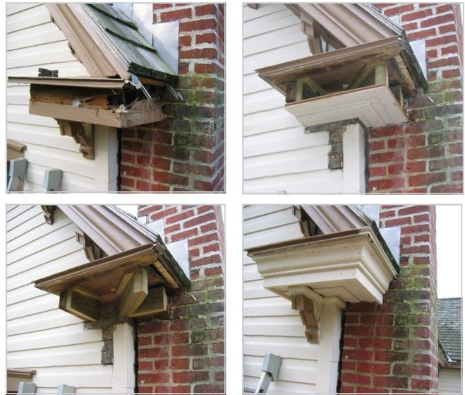
**Figure 22.** Sequence of restoration of a severely deteriorated cornice return. The crown molding was custom-cut for the project, a procedure that requires scheduling but does not add significantly to the repair cost.
