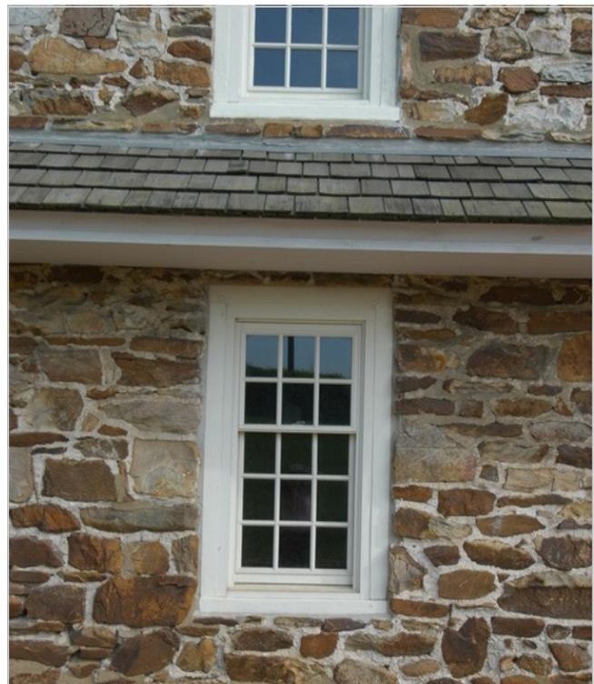
**Figure 47.** *Standard size vinyl replacement windows fitted to window frames by means of wood filler strips destroy the original proportions of the windows and are not recommended.*
