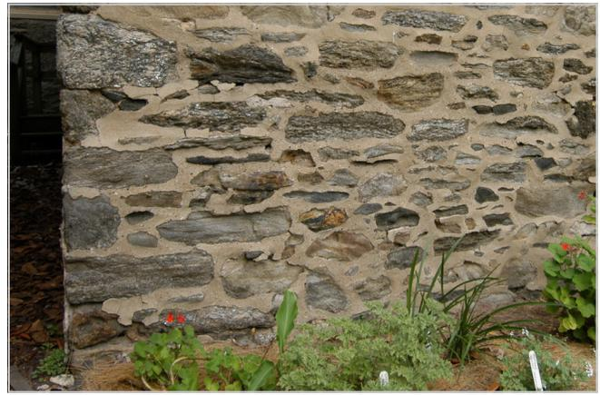
**Figure 31.** Overly-hard Portland cement mortar restrains the expansion of permeable stone masonry and results in the delamination (loss) of the face of the stone.
