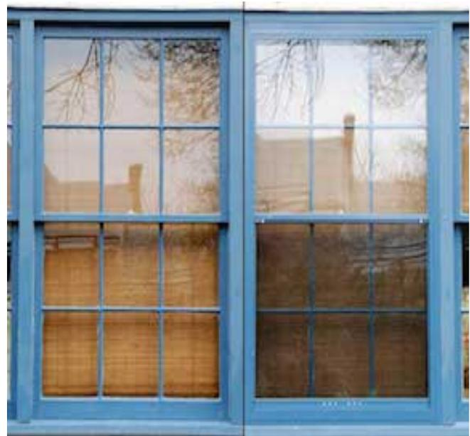
Figure 48. *Three-track Storm Window*
