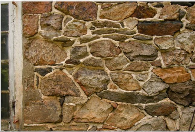
**Figure 30.** Detail of eighteenth century pointing. The most common joint profile type for rubble stone masonry was the raised ridge joint.
